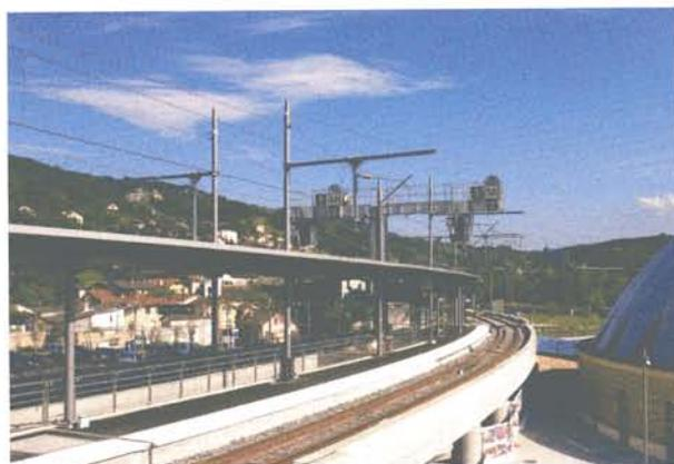
*Conversion of 1 500 V DC electrified lines to 25 kV 50 Hz single-phase current: the case of the Bellegarde – La Plaine – Geneva line*
