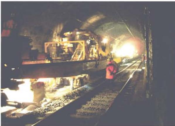
*Repairing the railway platform of the tunnel of Livernan*
