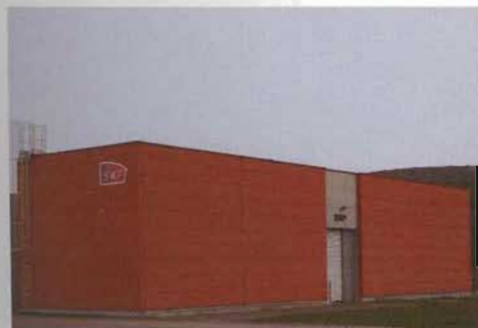
Maintenance in Operational Condition (MCO) of signalling equipment
