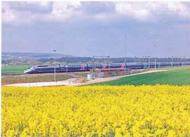
High-speed line project LGV+ Paris Lyon
