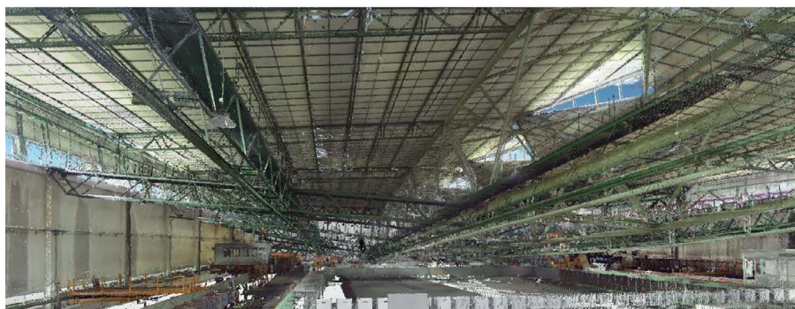
Exterior, axonometric and interior views of the 3D point cloud of the roof of the CEPYC Maritime Experimentation Laboratory.
