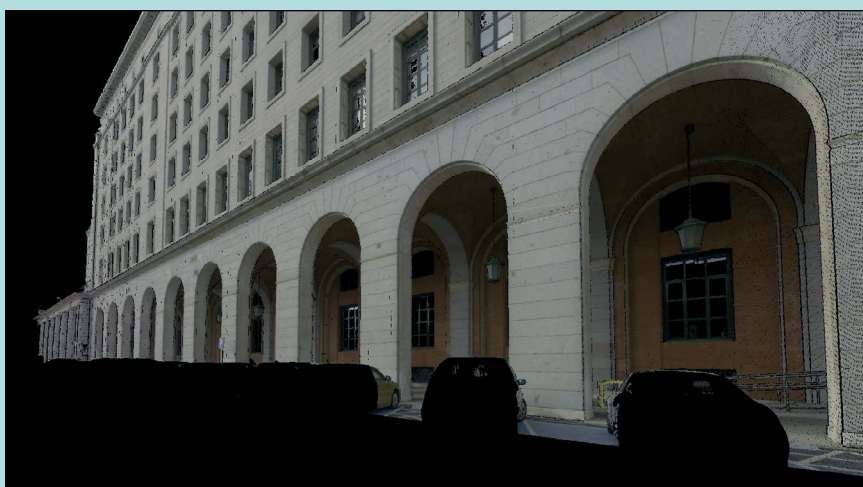
Point cloud of the façade of the Ministry of Transport and Sustainable Mobility.
