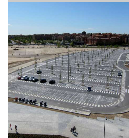
Fig. 7. Car park at the Wanda-Metropolitano stadium.
