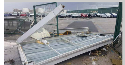
Fig. 10. Property damage after the tornado. November 2021.
