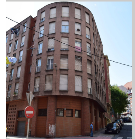
Fig. 2. Renovation of the façades and roofs of 14 entranceways in the El Patronato district.
