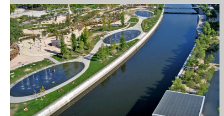
Fig. 4. Image of the completed Madrid Río Park.
