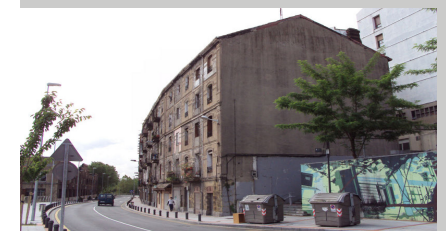
Fig. 4. Txabarri. Numbers 25 to 31 - before the work
