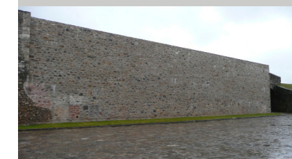
Fig. 9. Photograph of part of the walled enclosure of the Citadel of Jaca, Huesca.
