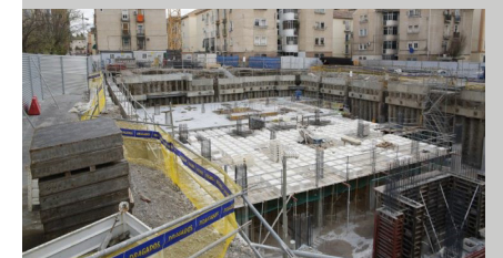
Fig. 4. Work in the Santa Adela neighbourhood.
