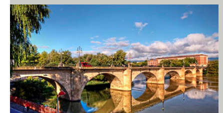
Fig. 3. Photograph of the stone bridge in Logroño, a restored section of the Way of St. James.
