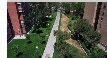
Fig. 5. Permeable paving and underground pipes in Gomeznarro Park.
