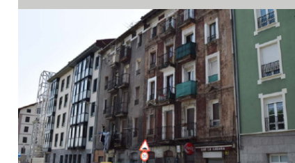
Fig. 9. Façade of a block in Sestao Berri.
