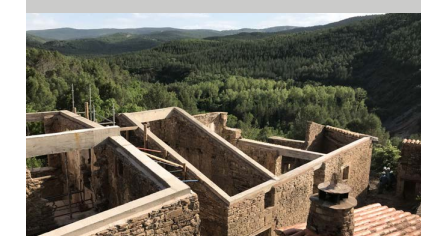
Fig. 5. Structural reinforcement with concrete beams.
