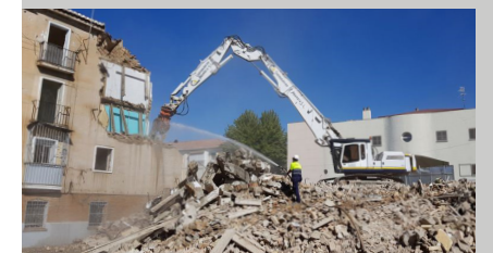
Fig. 3. Demolition of buildings covered by the action.
