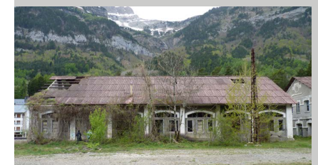
Fig. 3. Sanitary building. Before photo.
