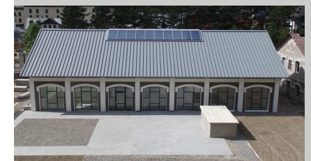
Fig. 4. Refurbished sanitary building, Reception Centre for Pilgrims.
