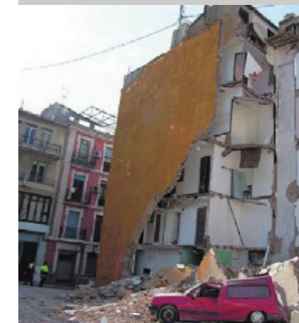
Fig. 7. State of a property in Calle Sant Mateu, after a house had collapsed.
