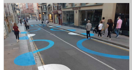
Fig. 11. Minor work on the asphalt in Calle Sagasta.
