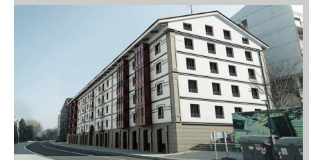
Fig. 5. Txabarri. Numbers 25 to 31. Photo montage of the refurbishment work.
