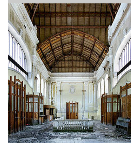
Fig. 7. Old station foyer, future hotel.
