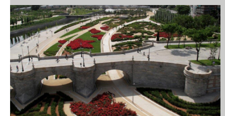
Fig. 6. Image of Madrid Río Park, Bridge of Toledo completed.
