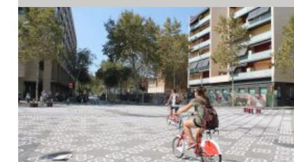
Fig. 9. Image of the work done.
