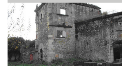
Fig. 8. Photograph of the Palace of Riva-Herrera, Cantabria, prior to its restoration and rehabilitation.
