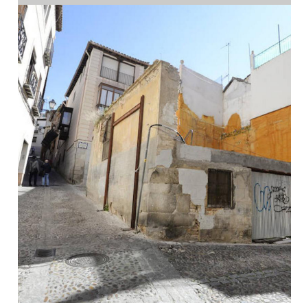
Fig. 7. Unoccupied building at the bottom of Cuesta de San Justo.
