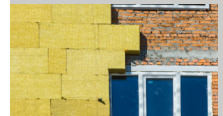
Fig. 10. Energy renovation of buildings.
