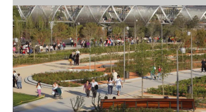
Fig. 8. Image of Arganzuela Footbridge.
