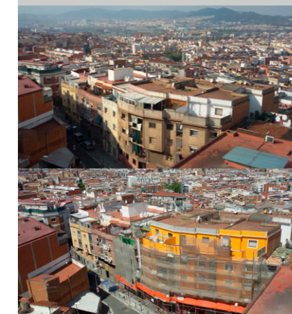
Fig. 7. Carrying out the rehabilitation of the façade.
