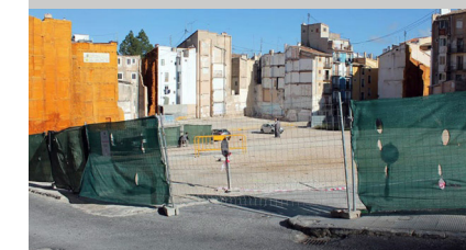
Fig. 10. Redevelopment of a plot of land for various social and recreational uses.
