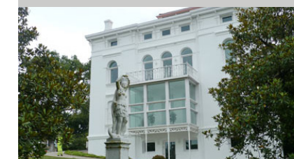
Fig. 10. Photograph of a façade of the White House on the Marqués de Valdecilla estate, Santander.
