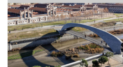
Fig. 11. Image of Matadero Footbridge.
