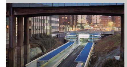
Fig. 6. Photograph of San Mames metro station.
