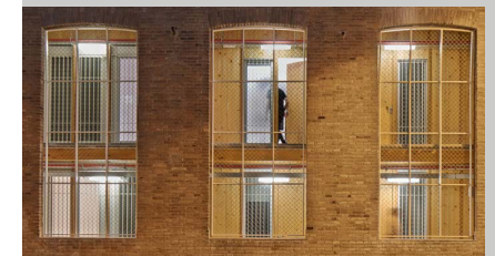
Fig. 11. Photograph of the façade.
