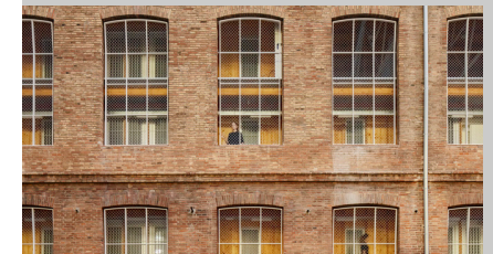
Fig. 9. Photograph of the façade.
