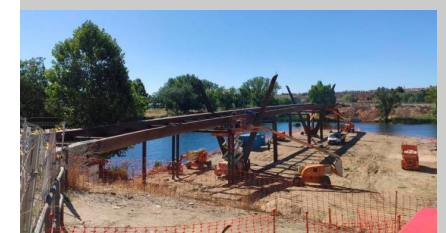
Fig. 5. Image of the footbridge being built.
