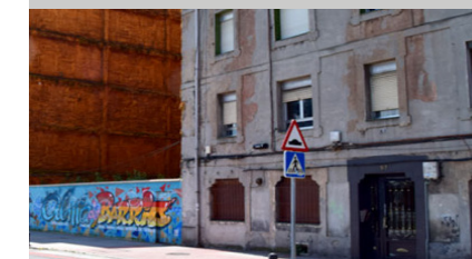
Fig. 10. Work began in July on the construction of 18 subsidised housing units in Txabarri.
